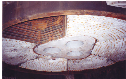
Figure 17. An electric furnace delta section shortly before operation.
